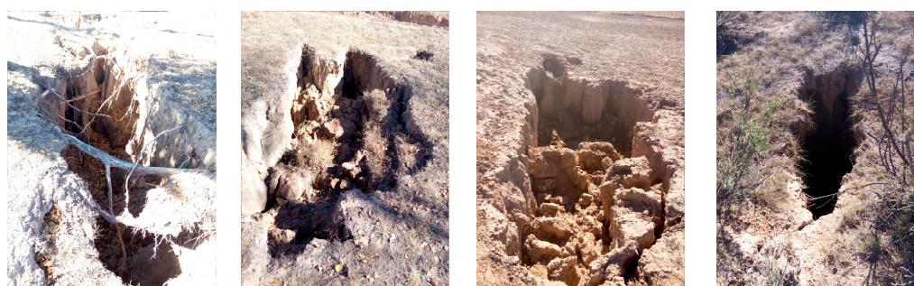
Figure 2. Ground fissure and collapse in the study area.
